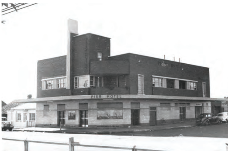
Fig 3.2.16. The Pier Hotel prior to re-building. By the time this photo was taken in the early 20th century the decorative detail had been removed. (BCHA)
