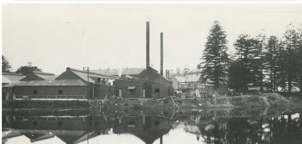
Fig 3.9.11 (top) Botany Pumping Station and the foreshores of Botany Bay with the Swinbourne and Stephen scouring works to its north (left) c.1893. Taken from Mudbank. (BCHA)
