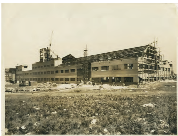
Fig 3.9.14 Construction of the Australian Paper Manufacturers Mill at Botany c.1935. (BCHA)
