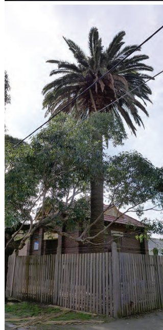
Fig. 4.4.23 the cottage erected for the SWSOOS engineer at 23 Byrnes Street adjacent to the line. By the 1980s it had been heavily altered, but the original Federation-style windows with sidelights remained. The property was known as ‘Twin Palms’ after the Canary Island Palms planted in its garden. (BCHA)
